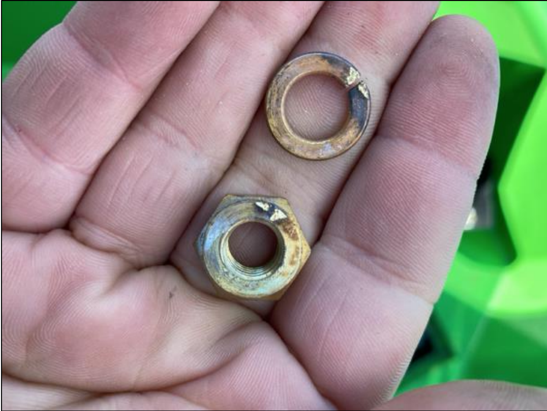
Photograph 12 – Nut and washer found loose on negative bow thruster terminal showing signs of arcing/excessive heat.
