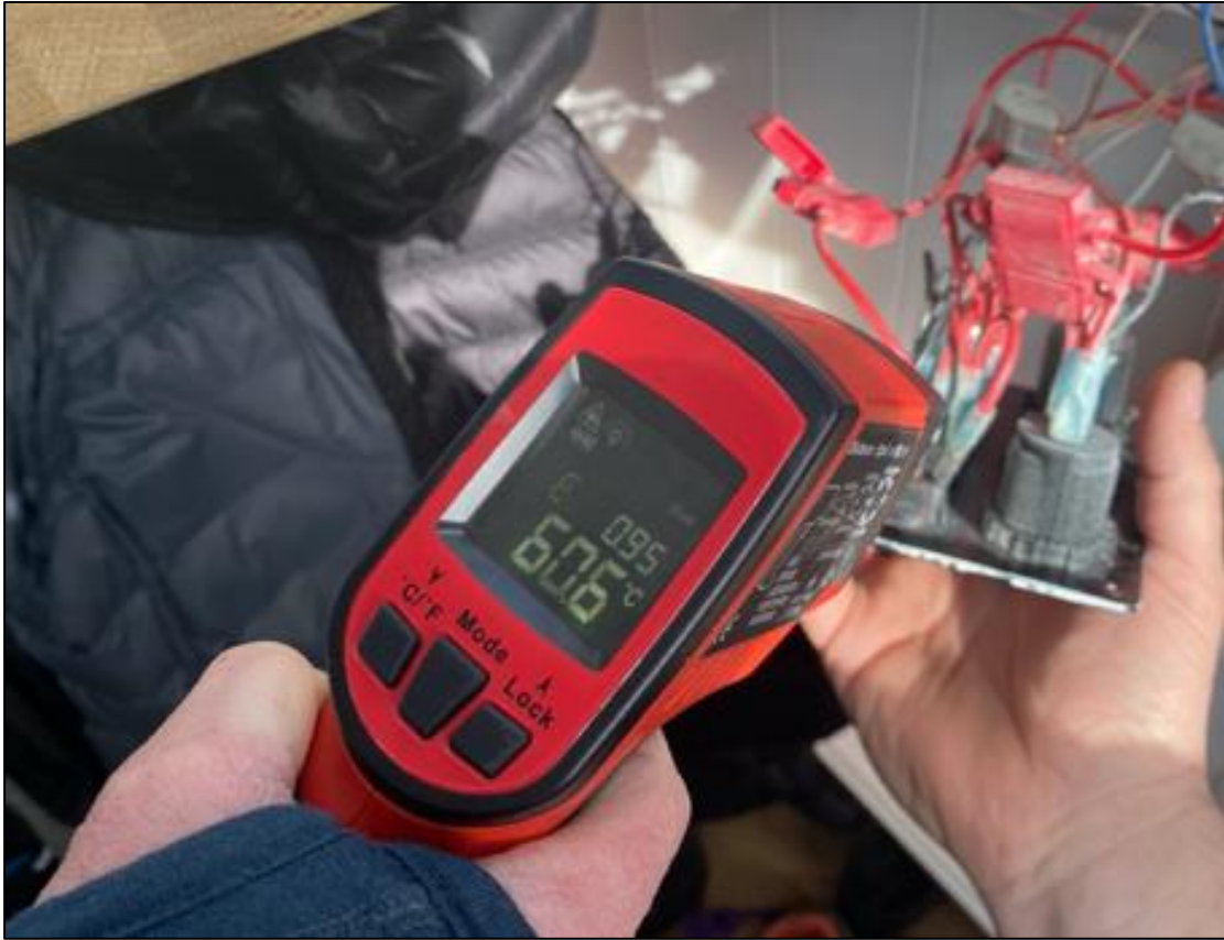
Photograph 17 – Switch showing a temperature of 60.6°C after 60 seconds of operation.
