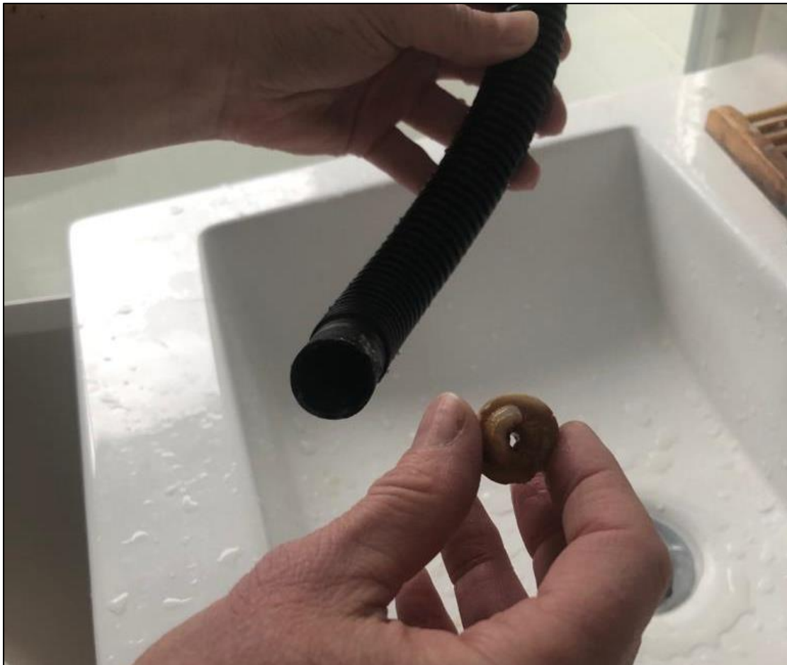
Photograph 20 – Silicone sealant found by owner blocking urine pipe.
